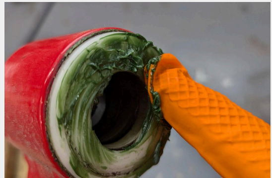
Figure 4: Apply grease
