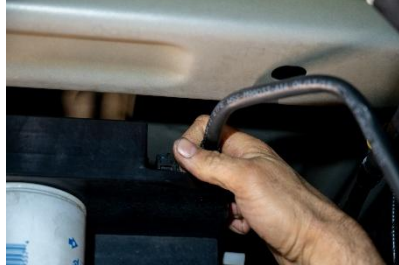
Figure 20: Reinstallation of fuel return line.
