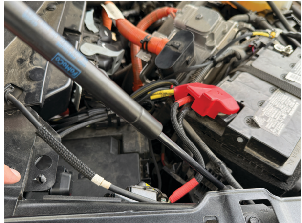
Fig. 79: Reinstall the cover and tree plug onto the 12V fuse block. Drill a hole to install the fuse block.
