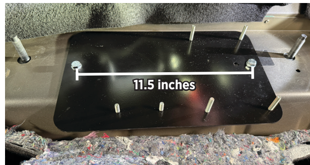
Fig. 51: Bracket and hardware installed.
