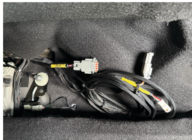
Fig. 87: CAN harness “Touchpoint” branch, not in use.
