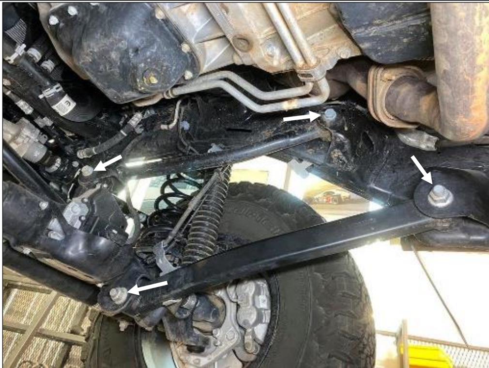
Figure 5: Passenger Side Control Arm
