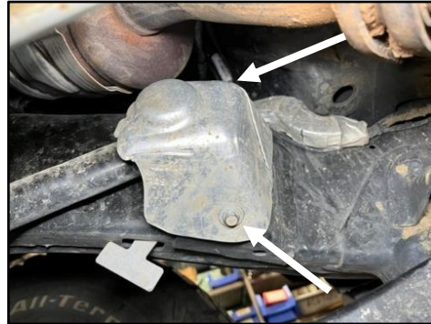
Figure 2: Passenger Side Heat Shield
