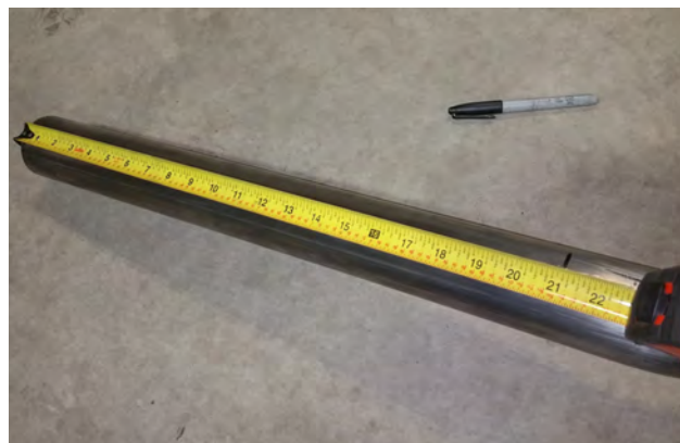
Detail 10a: 2 Doors only. Mark and cut 21" from mid pipe inlet.
